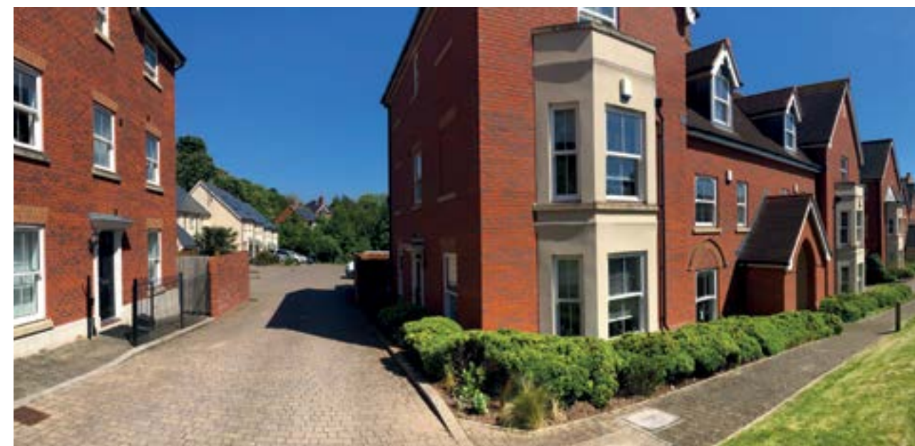
Affordable housing seen at the rear forms part of the Cyprus Gardens development
