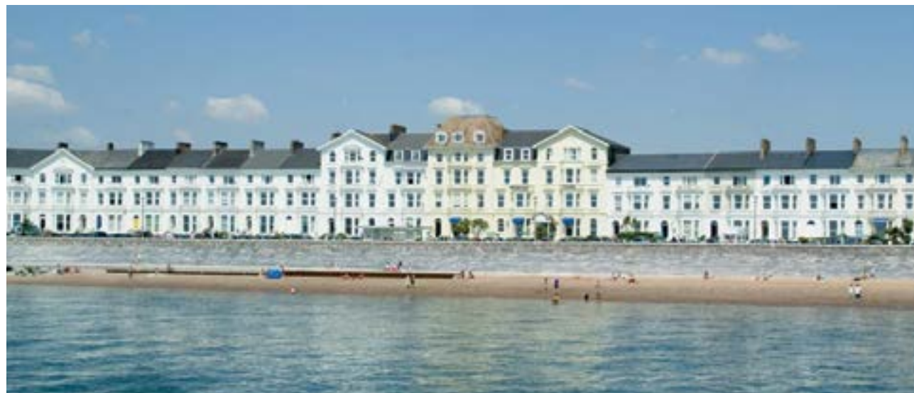
Smeaton's sea wall finished 1842
