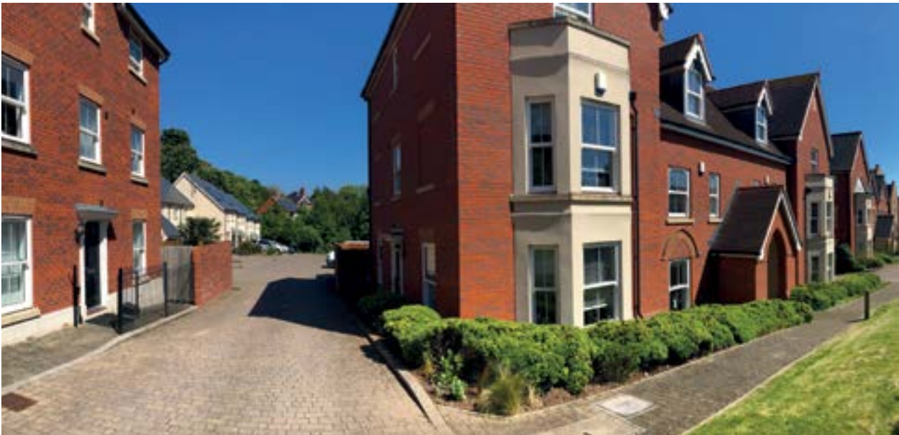
Affordable housing seen at the rear forms part of the Cyprus Gardens development
