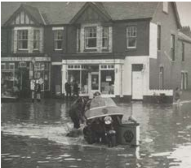
Junction of Hartopp Road and Exeter Road 1960
