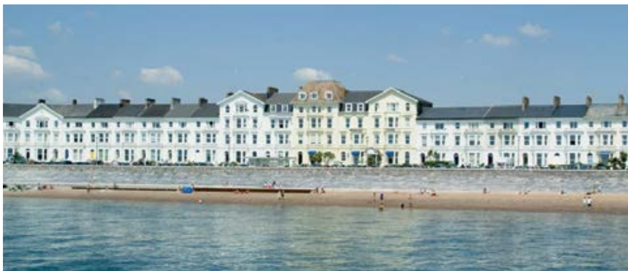
Smeaton's sea wall finished 1842
